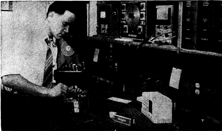
Fig. 1. Fixing a table-model radio. A few simple measurements with a multimeter locate the bad part, after which replacement with a high-quality new part is easy. (Centralab photo)
